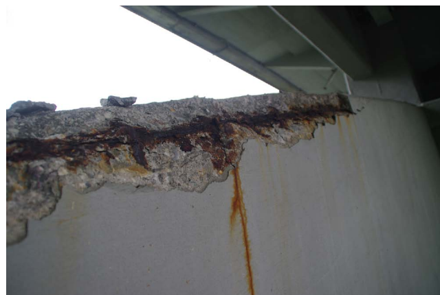
Figure 7. Example of damages to the arches
