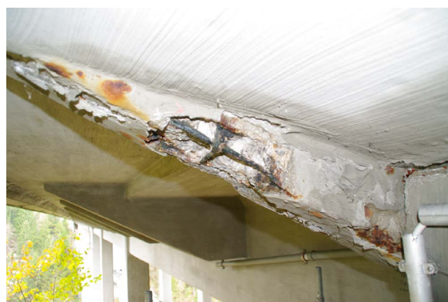
Figure 8. Damage to the console of the cantilever slab
